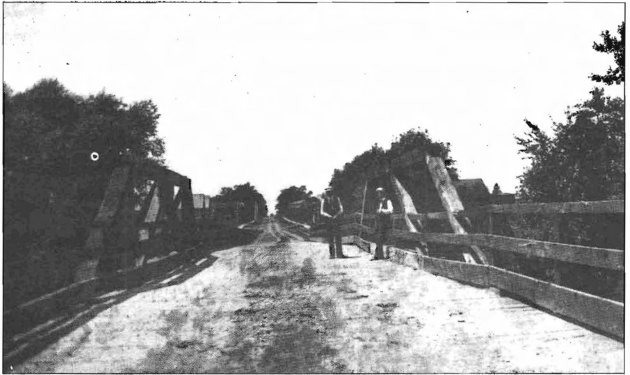
Photo (taken about 1910) showing the bridge across the Des Plaines River.
